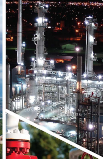
MONTANA DAKOTA UTILITIES BILLINGS, MT
